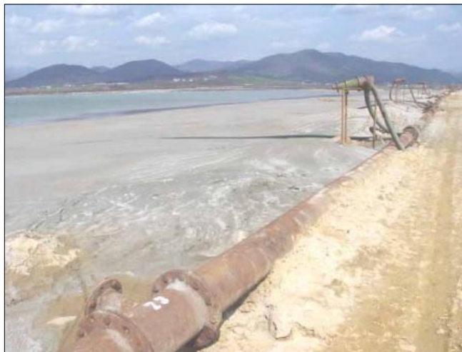
The Aurul dam, with hydrocyclones and the ‘beach’
