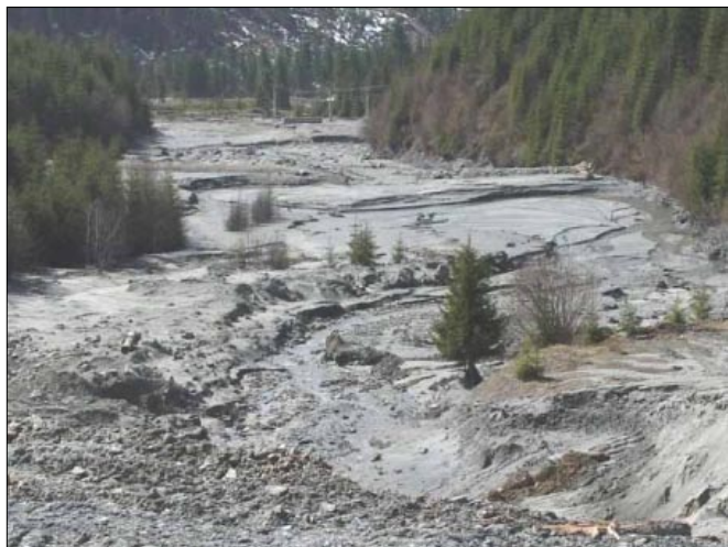
View from top of main dam at Baia Borsa, showing overflow sediments
